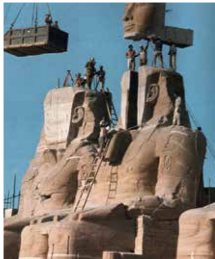
Premeštanje hramova u Abu Simbelu zbog izgradnje asuanske brane, 1968./ Relocation of the temples in Abu Simbel due to the construction of the Aswan Dam, 1968
